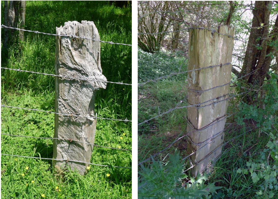
Figure 8. Examples of old fence posts near the Wēiti Stream. The post on the right is split totara.
